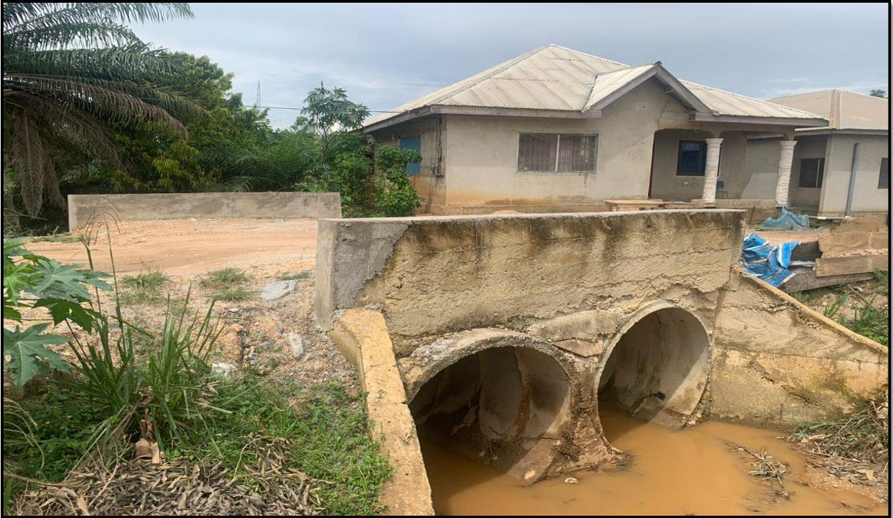
**Constructed 8m Double 1800mm Diameter Pipe Culvert at New Nyamebekyere (MPCF)**
